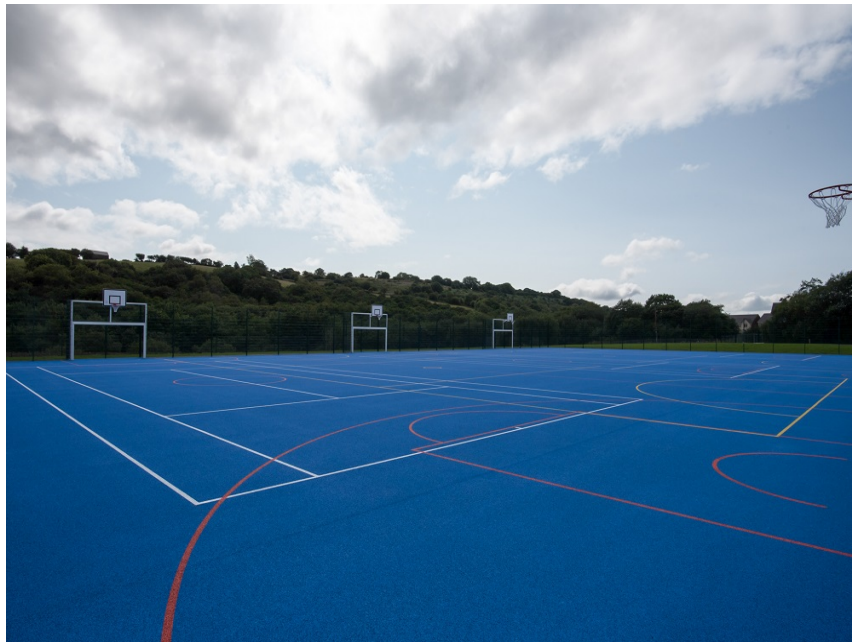
Example of MUGA servicing Tonyrefail Community School.
